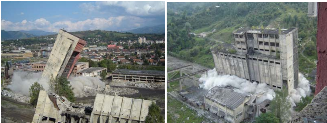
Demolition of Dalja Mine Unit
