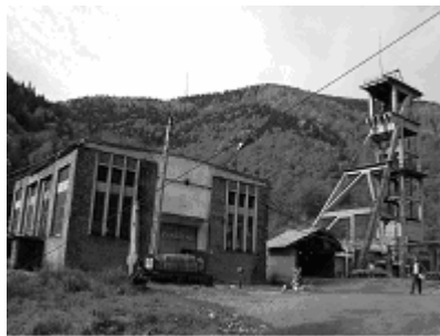
Fig.2. Extracting installation „ Auxiliary well no. 2 “
